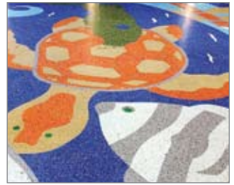
Glass flooring installation at Jacksonville International Airport
