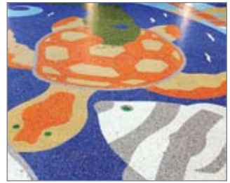
Glass flooring installation at Jacksonville International Airport
